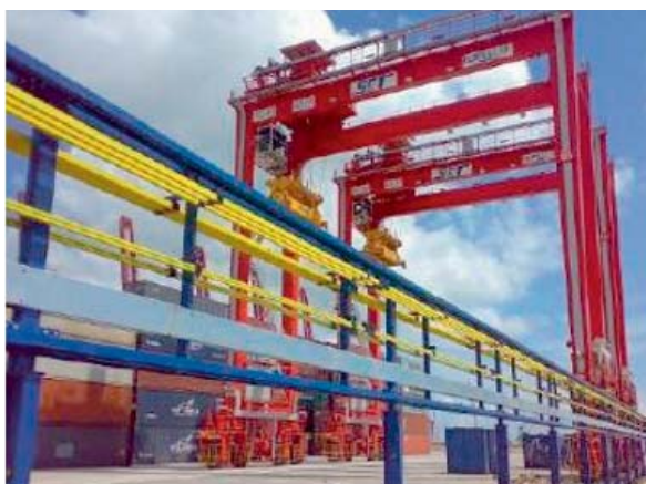
Figure 4 Common type of Conductor Bar (or Bus Bar) RTG Electrification System
