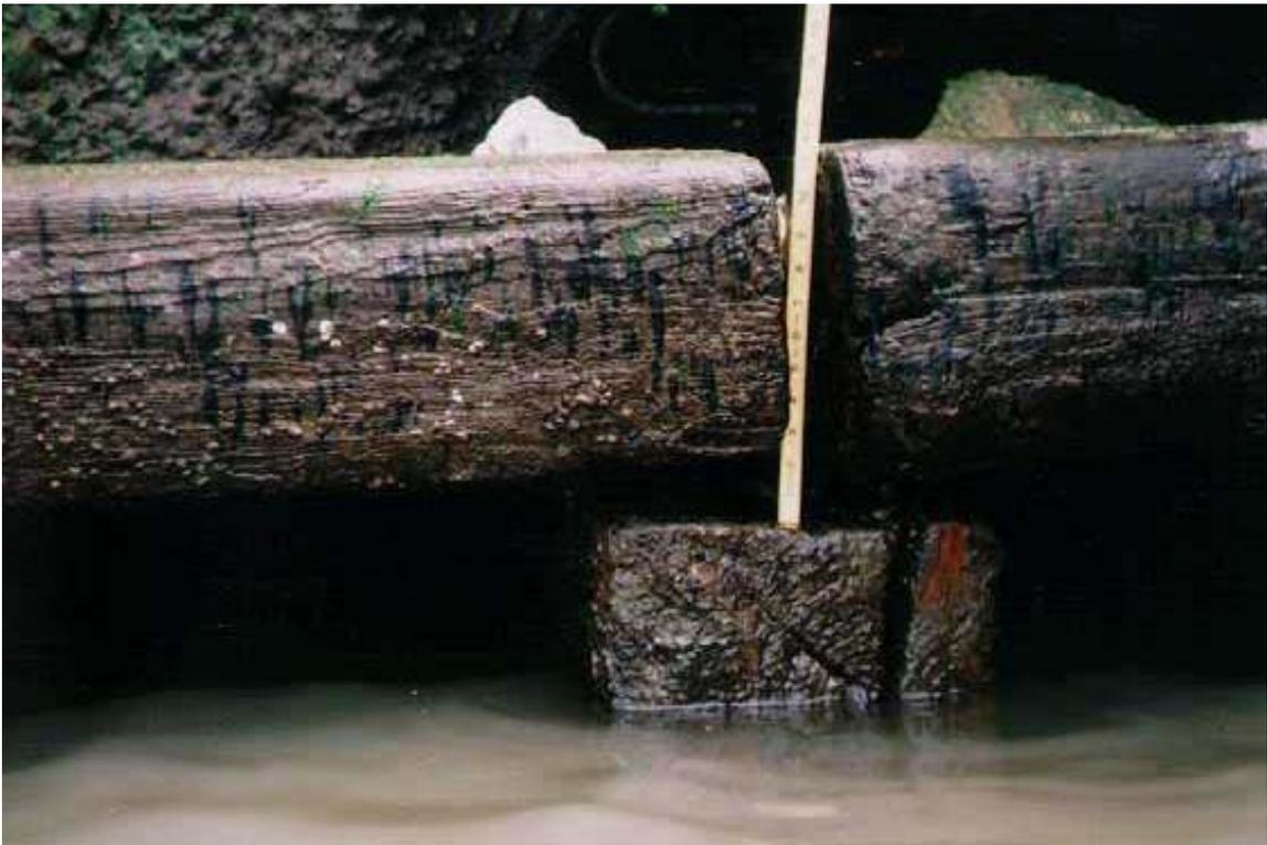
PHOTO 7-2. Non-bearing timber pile cap at offshore end of bent.
