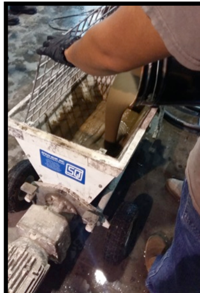
Bombeo del Epoxy grout
